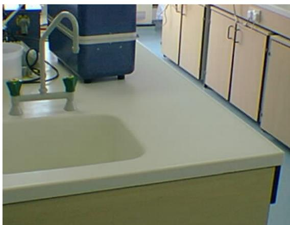
**Figure 1** Photograph showing a suitable lipped Corian® bench and integral sink
